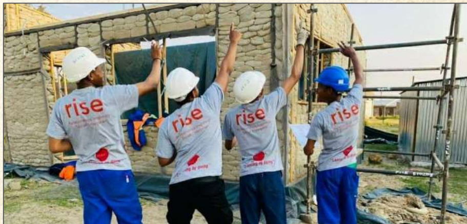
Fellows construct the Seboka Primary School kitchen
