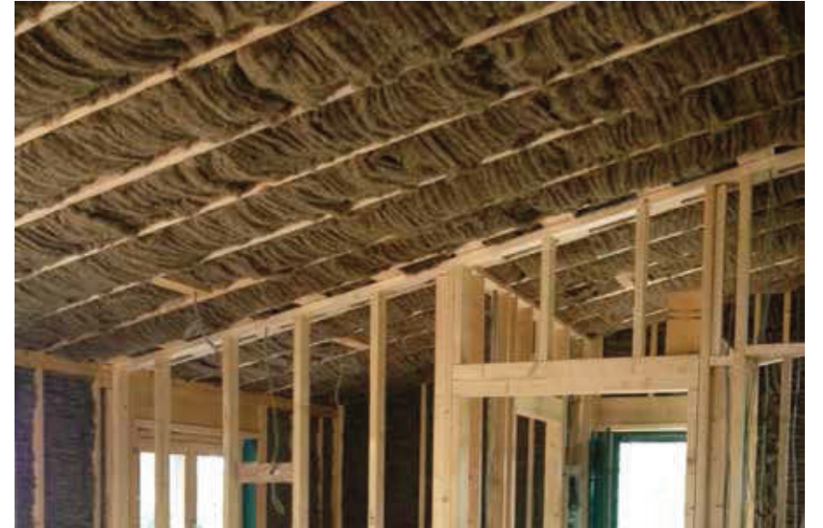
Sheep wool insulation in the ceiling.
