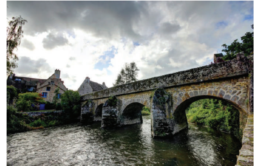
Sarthe River Bridge in Saint Ceneri le Gerei, 500 AD, France. Hemp mortar was used for construction
