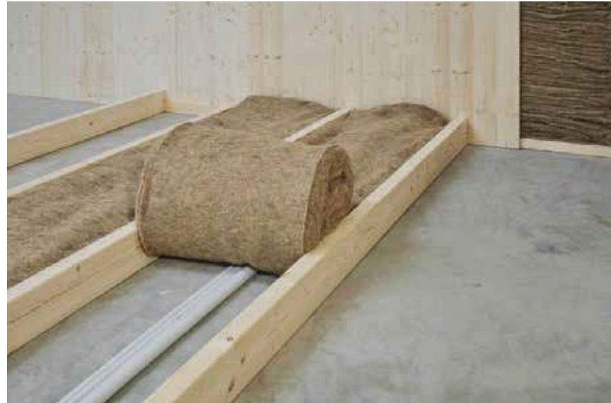
Sheep wool insulation for the floor.
