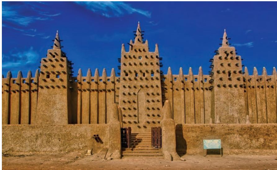
Located in Mali, the Djenne mosque was constructed in the thirteenth century. It is the largest mud brick building in the world. (Adobe bricks)
