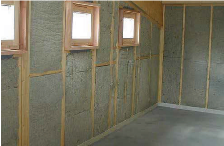
Wool insulation in the walls.
