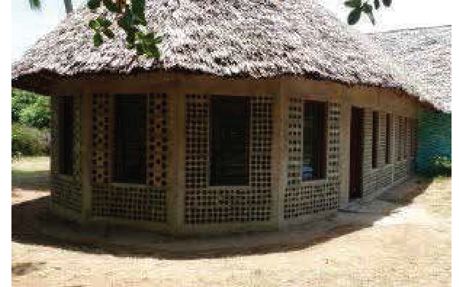
Glass bottle construction in Wamatu
