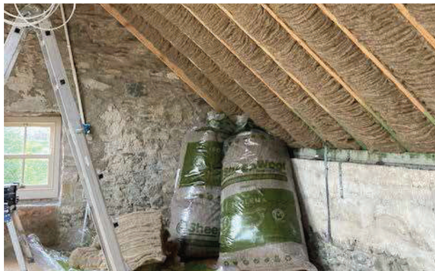
Sheep wool insulation in the attic.
