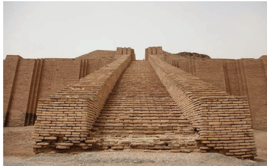
The Great Ziggurat of Ur of ancient Mesopotamia c. 2100 B.C.E. Constructed of mud brick covered with baked bricks laid with bitumen
