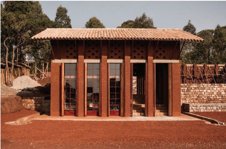
Children's library in Muninga in Burundi, built from compressed earth blocks. Designed by BC Architects
