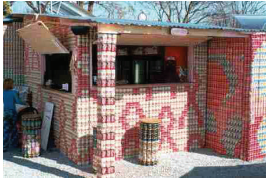
Soda can structure in Lesotho, built in 2002, designed by Michael Hönes
